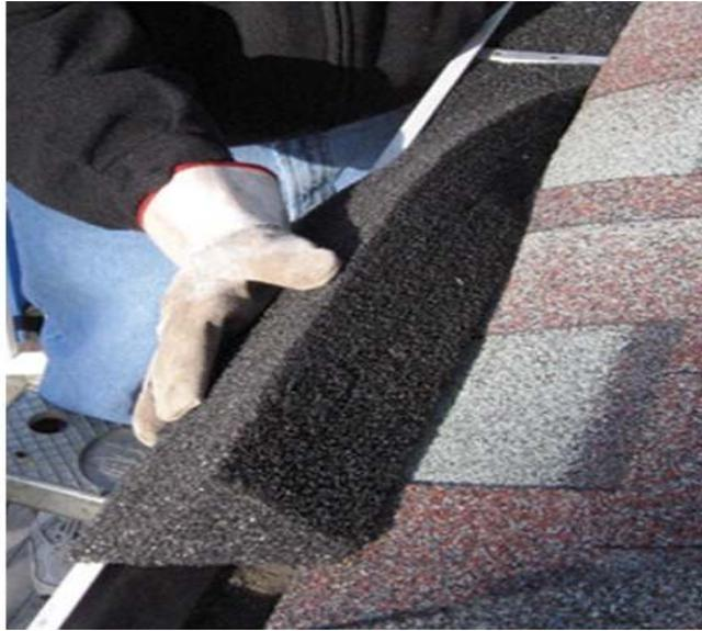
Foam Filter Inserts are screwed to the roof or the gutter lip. They slide into the gutter under the spikes or hangars and can be installed into hidden/built in gutters.
